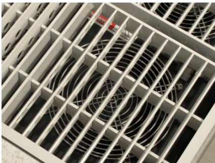
4 x Redundant Energy Efficient EC Fans with 0-100%
